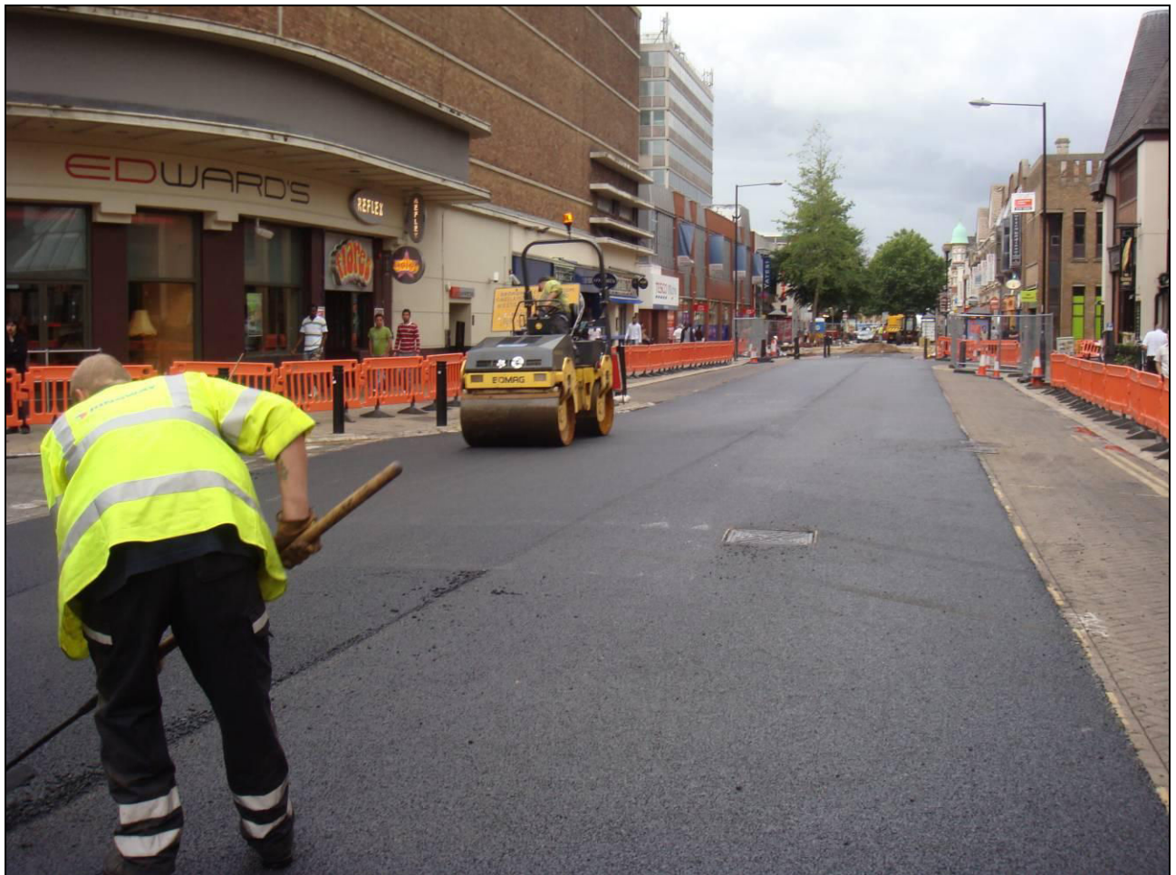
Figure 6 Resurfacing of Broadway 2009
