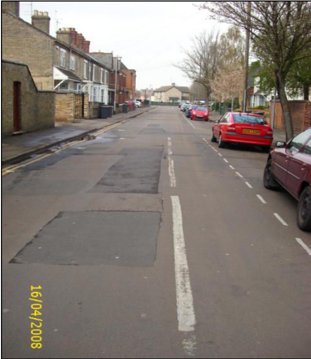
Figure 7 Manor House Street before Resurfacing
