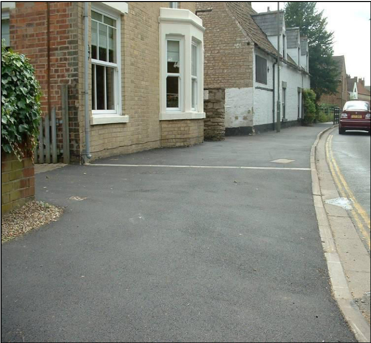
Figure 18 Church Street Werrington after Slab Replacement Scheme
