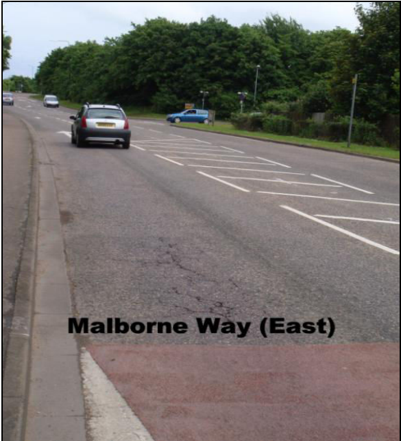
Figure 4 Malborne Way prior to Resurfacing
