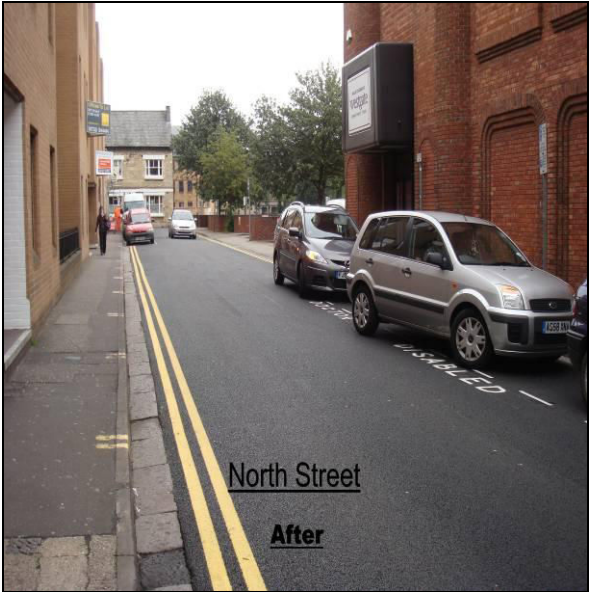
Figure 3 North Street after Resurfacing
