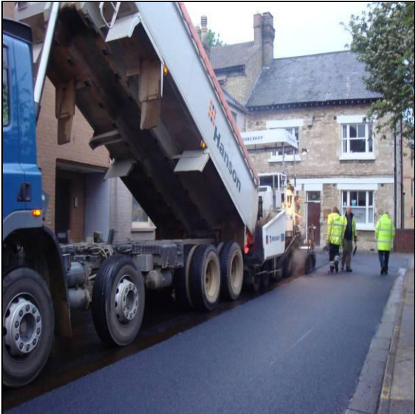
Figure 2 North Street during Resurfacing
